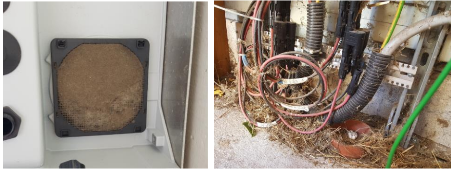
Dirty Inverter filter: derating in power
