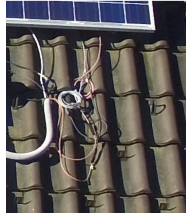
Poor wiring
